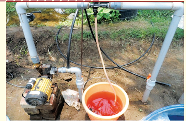
Fertigation through Venturi
